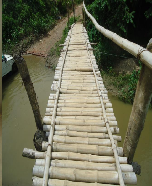
Bridge connecting Korbong village
